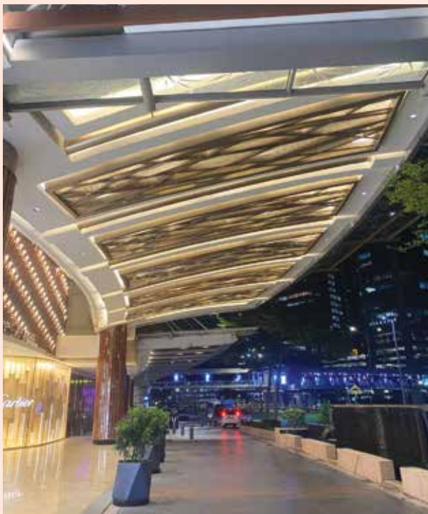
Replaced the West Deck canopy lighting for improved visibility and safety
