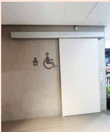
Installed automated sliding doors for Disabled-Accessible Toilets
