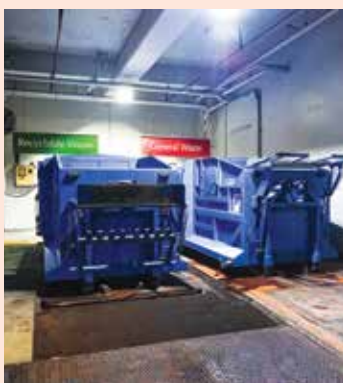
Upgraded refuse chambers at Loading Docks A and G
